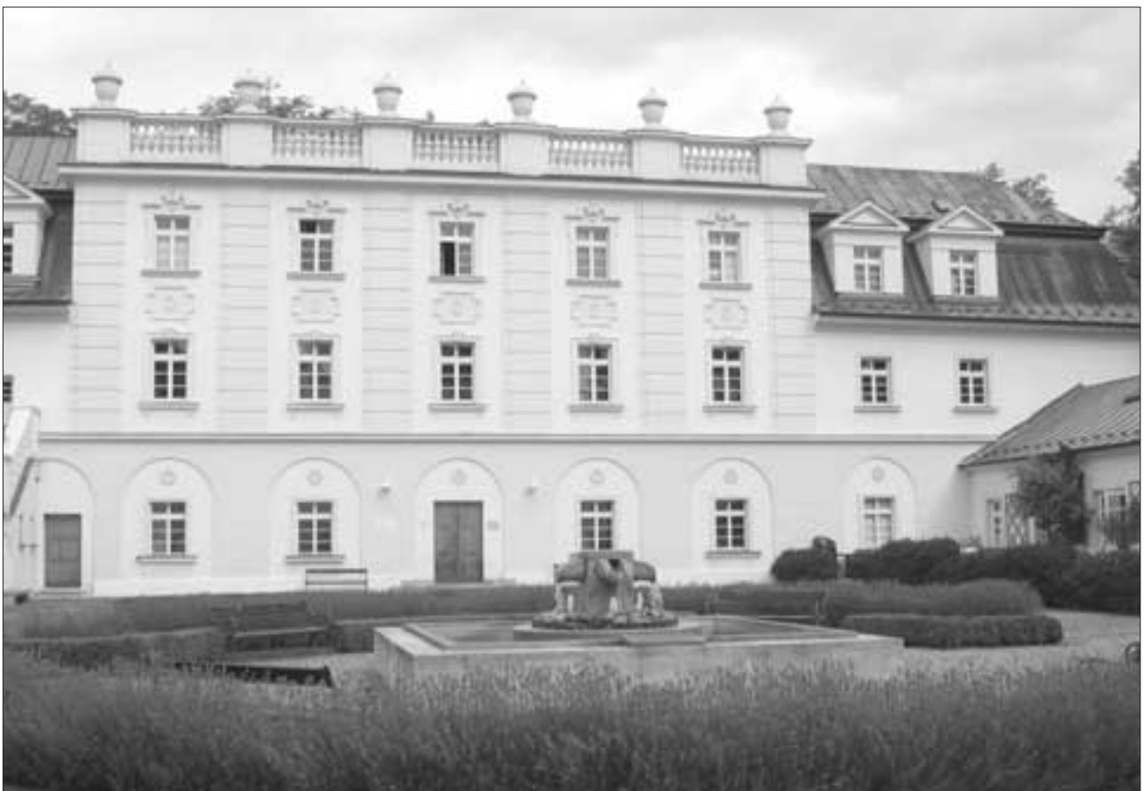
IBTS library main entrance
